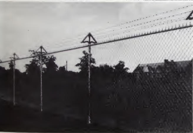
This Non-Climbable Fence also has the arms arranged in an A-shape. Even if an intruder should get across he would have a great deal of difficulty getting out quickly.
